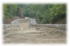
Section 60.3.4 (from Petritsi Interchange to Promahonas). The project consists of flood control works design, in one of the major interstate rivers of Greece (Strymonas river), with flood flux estimation of 3.500m<sup>3</sup>/sec, in order to protect the Egnatia Highway network, passing by the river on the narrow border passage.
